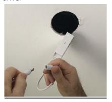
Make sure both side of the connector are pushed-in and turned
