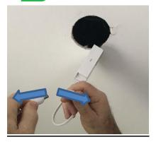
3. Pull down the driver until the mains plug is visible
